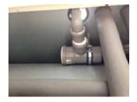
Fill the collection tank for the condensate hoses with a hydraulic seal.
