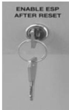
Figure 26: ESP activator lock and key
