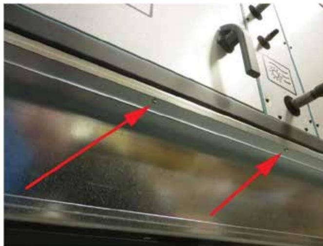
Figure 12. Base Frame Mounting
