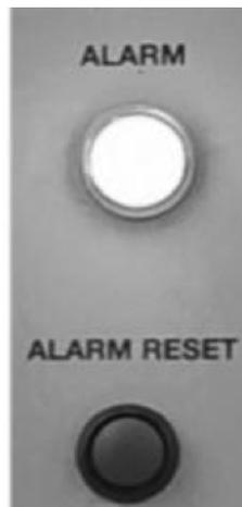
Figure 27: The alarm lamp and alarm reset button
