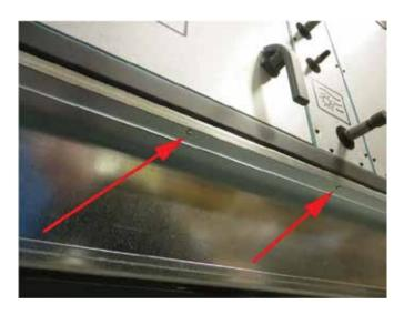
Figure 12. Base Frame Mounting
