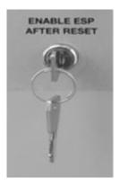
Figure 26: ESP activator lock and key
