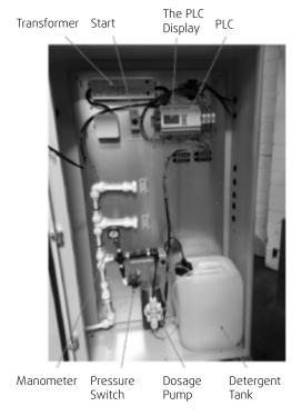
Figure 24: Internal setup of the Autowash system
