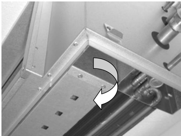
**4.** Placera hållare/ Place the droplet eliminator holder in position/ Halterung anbringen.
