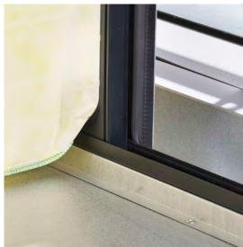
Check that the grey flexible profile on the vertical metal frame that holds the filters is without wear and damage and that the grey flexible profile is still sufficient for avoiding any air leakage between the closed inspection door and the frame that holds the filters.
