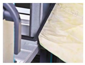
Check that the filters are pushed to the position where the vertical frames of the filter bags are closing fully to the flexible vertical lists in the air handling unit for avoiding any air leakage.
