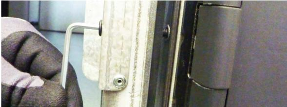
Insert the screw in the hole and tighten the screw. It might be useful to pull the sections fully together prior to tightening the screws.
