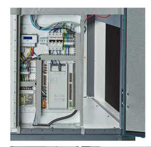
Cable entry is always in the bottom of the air handling unit
